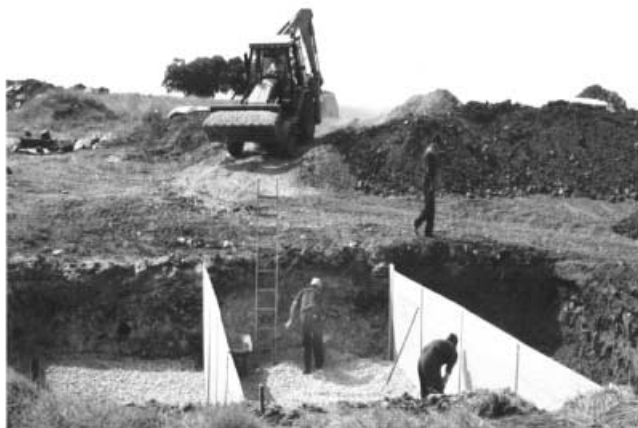
Figure 3. Construction of the experimental wetland
